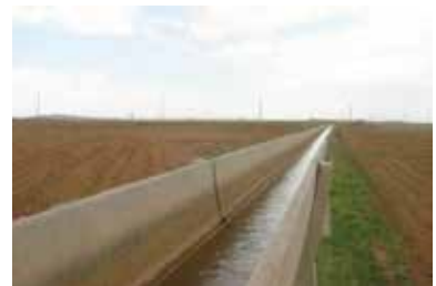
Figure 17.2. The Ataturk Dam, part of the GAP project in Turkey, diverts water from the Euphrates River (left). The main canal (middle) conveys water to the Harran Plain for distribution to individual fields (right).
