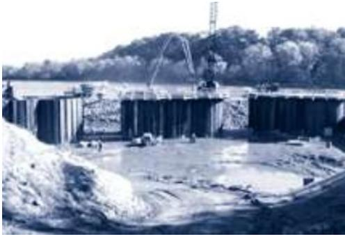
*Crews erect coffer dam cells as part of the fish passage facility at York Haven, Fall 1998. The construction will be complete in time for the spring shad run in 2000.*
