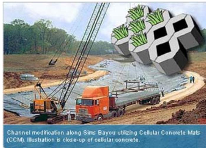
Figure 1. Example of articulating concrete block used at various sites.
