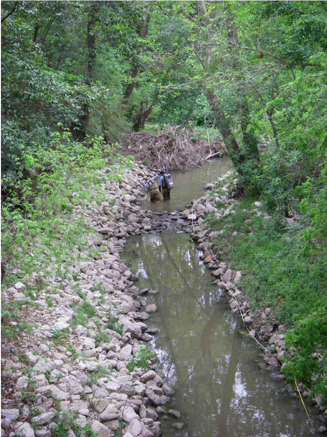
Figure 24. Rummel at the downstream Audubon Bird Sanctuary (RCB) on 4/1/09 after placement of rip-rap. View looking upstream.
