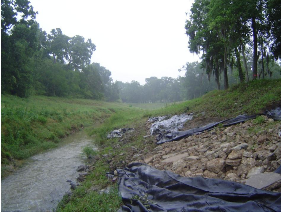
Figure 39. Cowart Creek Greenbriar site (COG) looking downstream showing partial rip rap shoreline with plastic liner. Rip rap was also deposited in stream to create minimal artificial riffle habitat. Photo taken in 2007.
