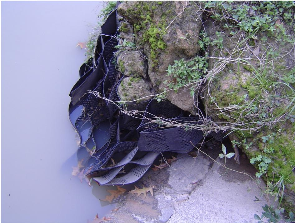
Figure 21. Close-up photo of corrugated plastic reinforced bank material at the Rummel Creek elementary school site (RCS). Photo taken 1/10/07.
