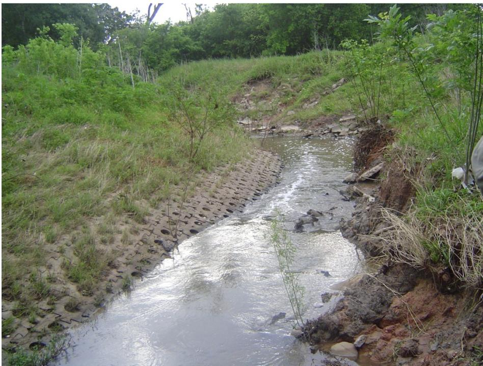
Figure 38. Cowart Creek Linson Site (COL) looking downstream showing articulated concrete bank and downstream artificial riffle habitat. Photo taken in 2007.
