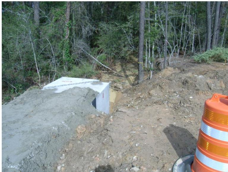
**Figure 66. Photograph of top view of new culvert installed near upstream of site 1 taken during stormwater sampling event 6 on October 10, 2011. (Source: hand held camera).**
