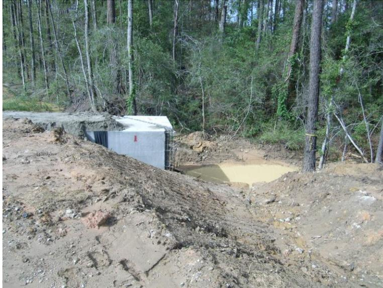
**Figure 65. Photograph of side view of new culvert installed near upstream of site 1 taken during event 6 on October 10, 2011. (Source: hand held camera).**
