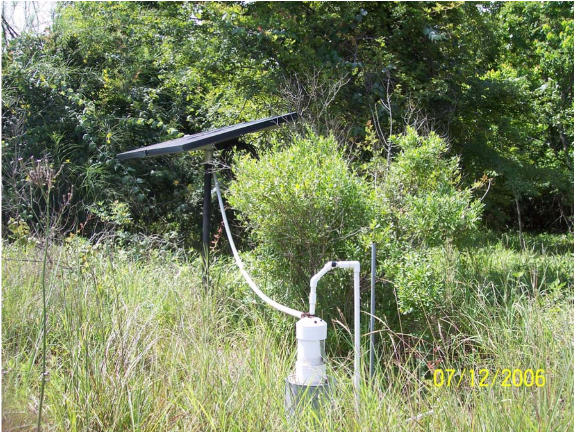
Figure 16. Solar powered irrigation system installed at the University of Houston Clear Lake campus.
