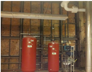
Expansion Tank Replacement
